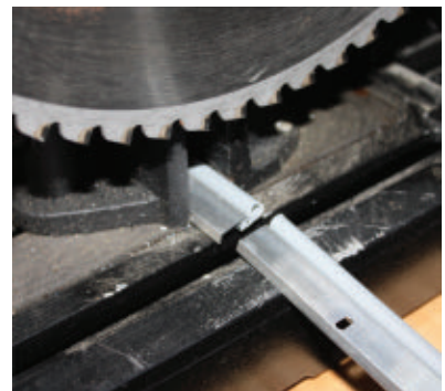
Cut the strip to length. I used a chop saw, but a hacksaw works best.
